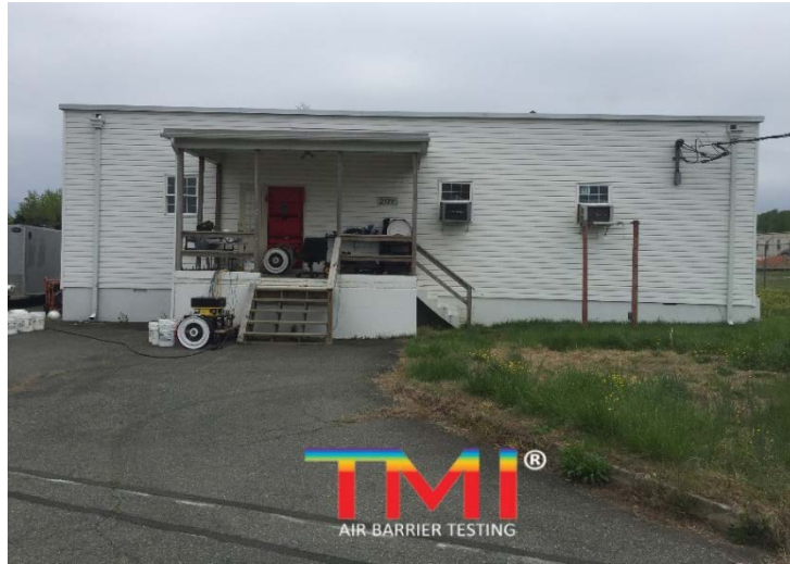
Figure 6. Office Building Sealed at Quantico MCB
